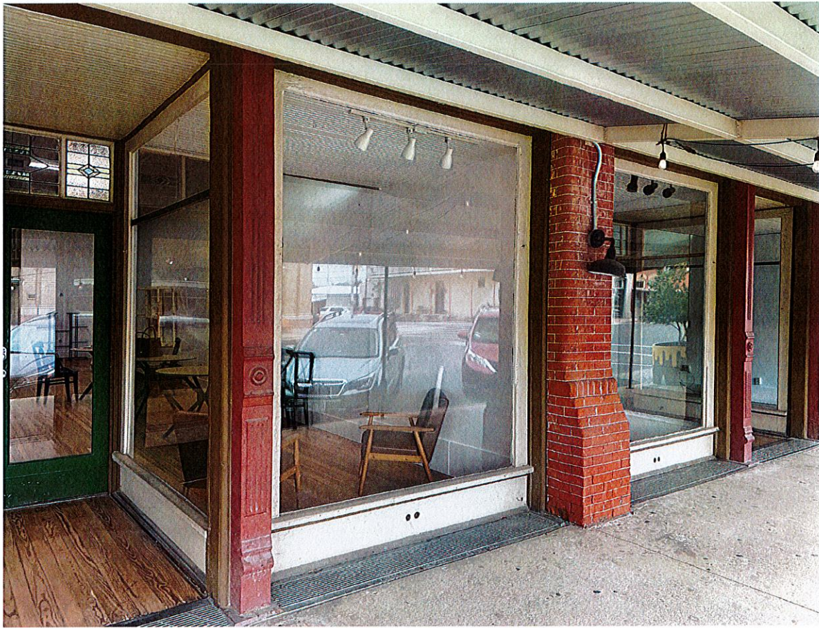
Location of painted window signage
