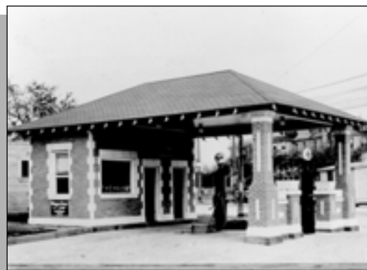
Figure 24: Many early Magnolia stations featured boxed columns constructed of brick, a hipped roof and exposed rafter ends.
