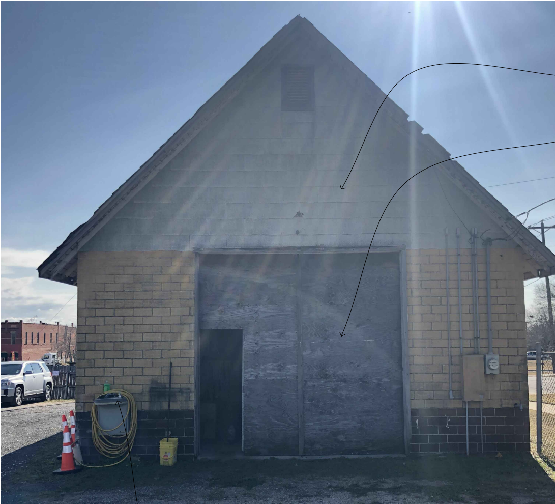
EPD YARD SIDE
