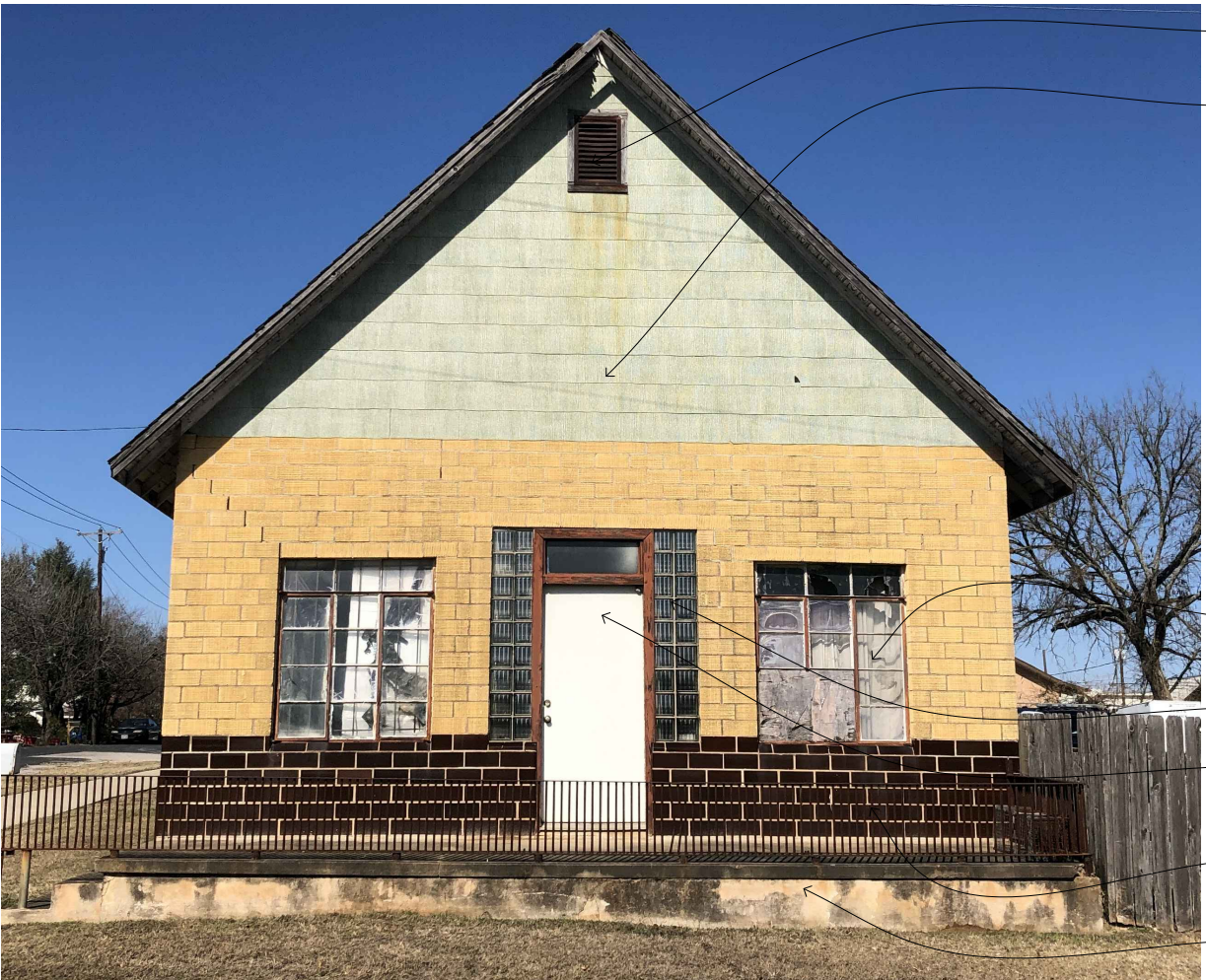
DEPOT STREET SIDE
