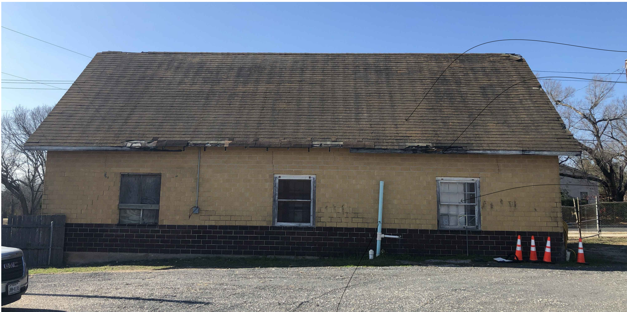
EPD YARD SIDE
