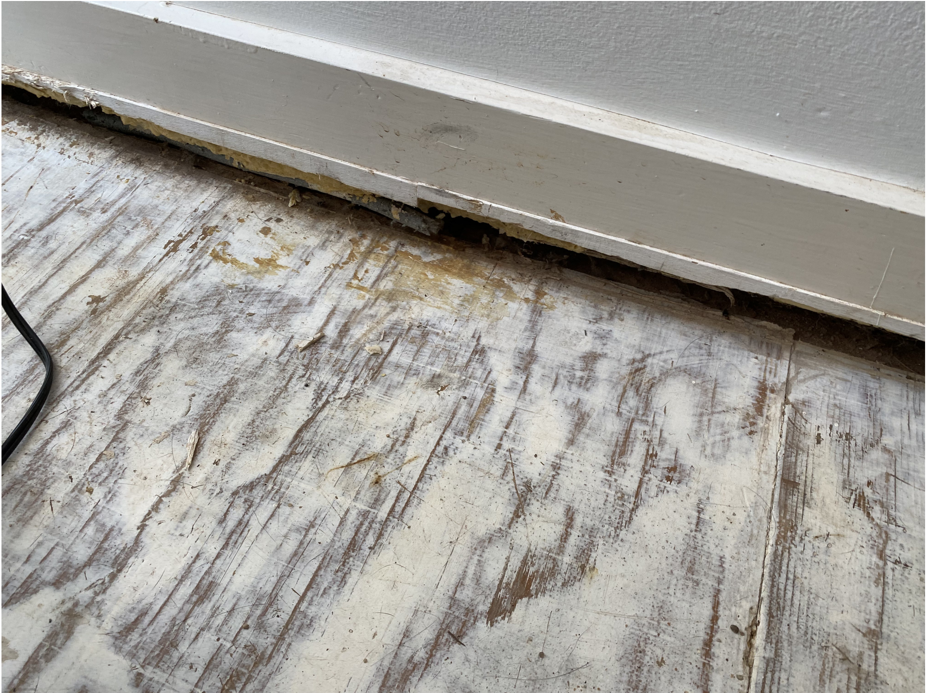
North wall closeup
