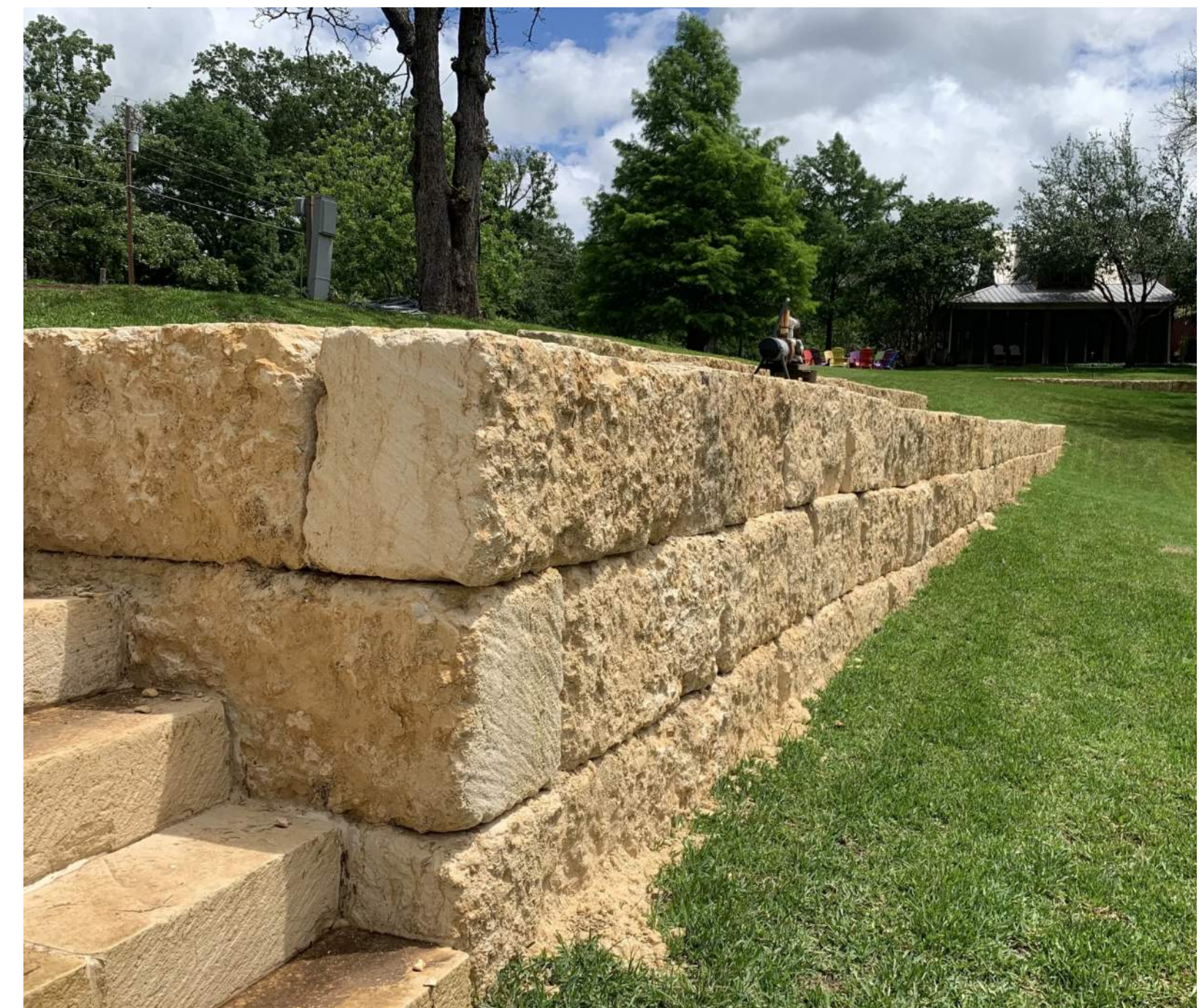
LIMESTONE BLOCK WALL
