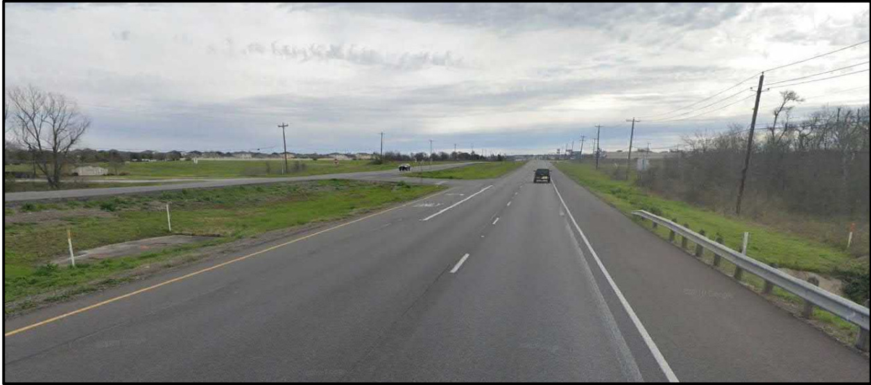
Figure 4 – US 290 and Western Sky Blvd Facing East
