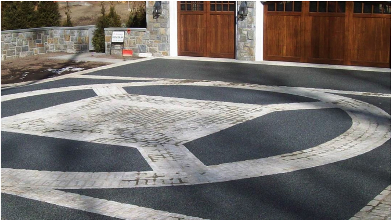
Example of flexible porous paving. This surface is permeable as opposed to impervious.
