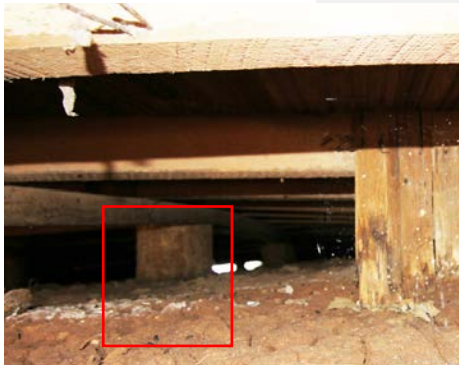
Foundation (looking northeast)
