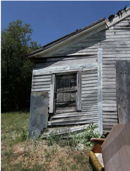
Metal Seam on East Elevation
