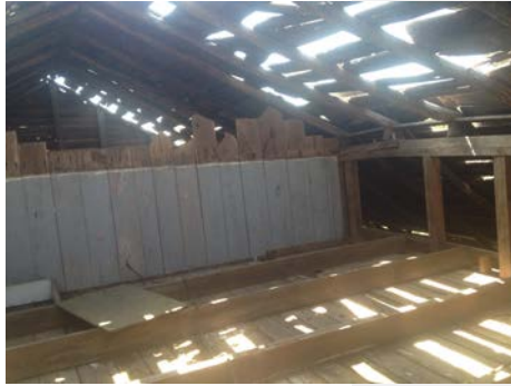
Roof Construction (looking southeast)
