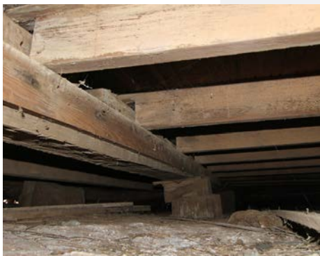
Foundation (looking northeast)
