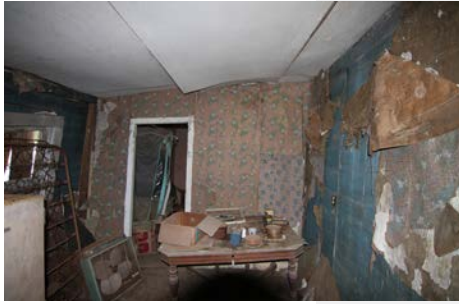
Ceiling in Kitchen/Dining Room (looking west towards the kitchen/bathroom addition)
