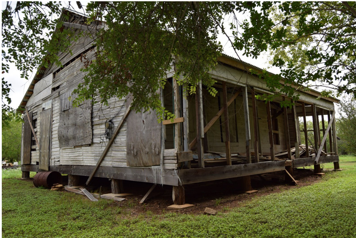
Photograph 2. West and south façades. Camera facing northeast.
