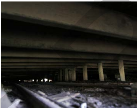
Foundation (looking northeast)
