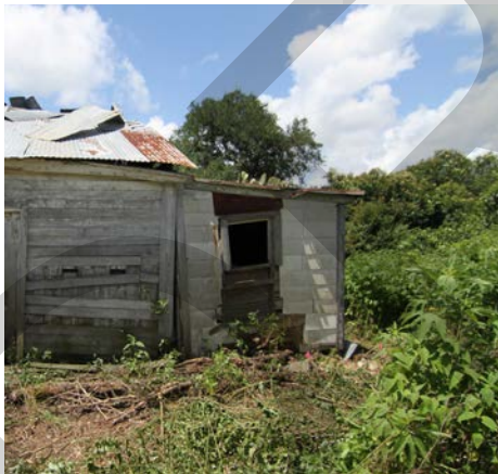
Northwest Corner (cacti on roof)
