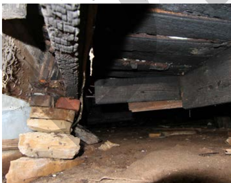
Foundation Under West Elevation (looking north)
