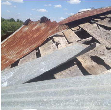
Roof Covering (looking east)
