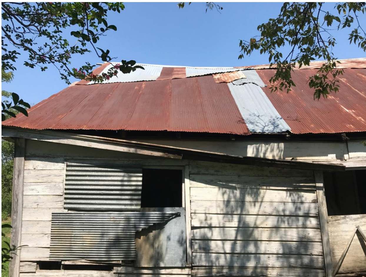
West façade detail
