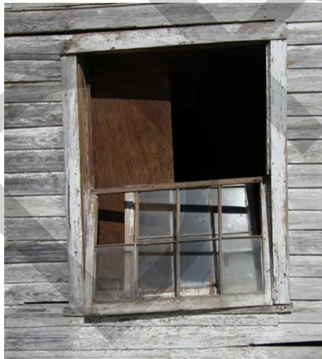
8 Over 8 Window on East Elevation (later addition)
