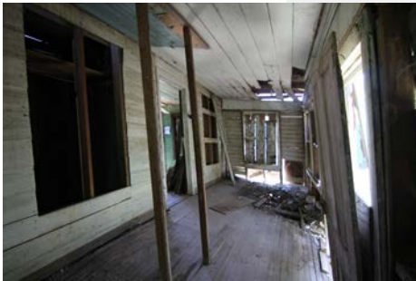
Porch (looking east)
