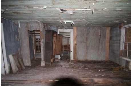
Dining Room (looking south)
