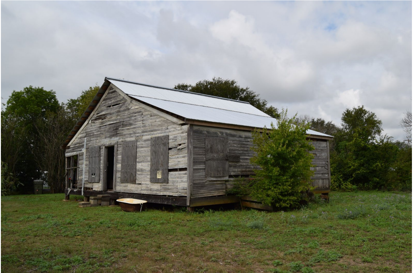
Photograph 6. North and east façades. Camera facing southwest.
