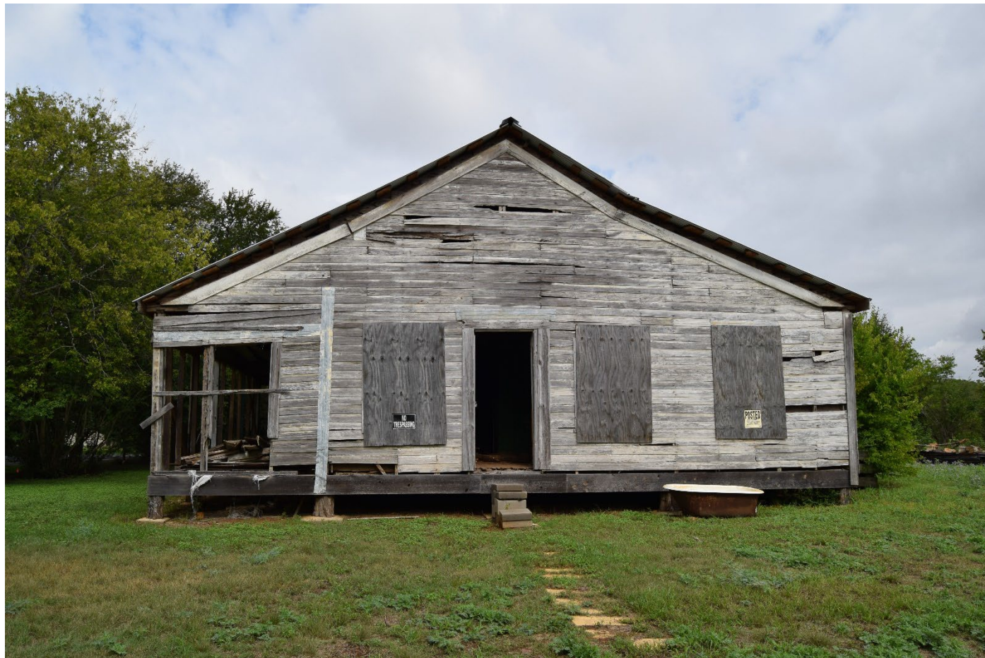
Photograph 5. East façade. Camera facing west.
