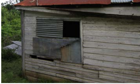
Varied Siding Sizes at Southwest Corner
