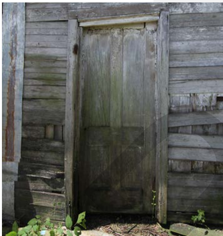
North Elevation Door
