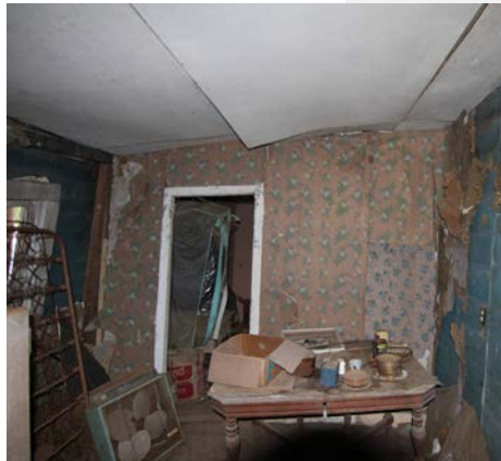
Kitchen/Dining and Back Bedroom Wall (looking west)
