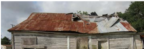
Roof Covering from North Elevation
