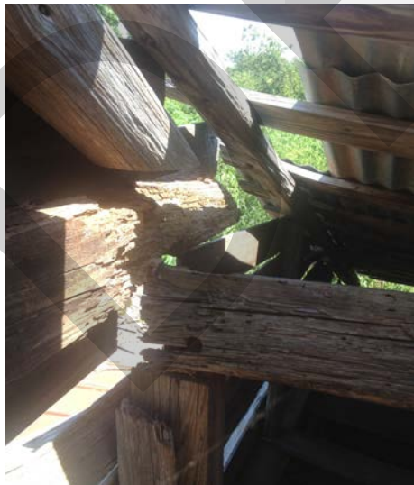
Roof Construction (northwest corner)
