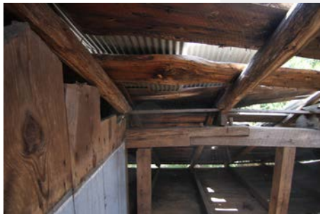
Roof Construction (looking south)
