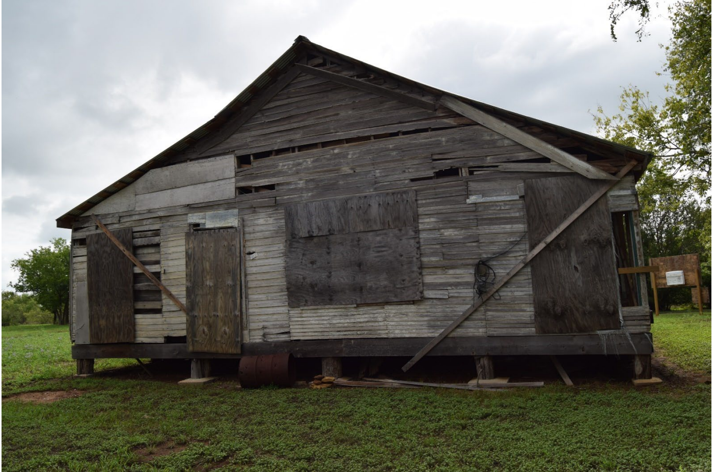
Photograph 9. West façade. Camera facing east.
