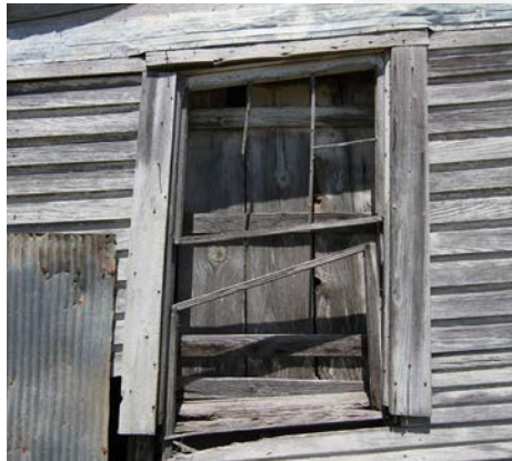
6 Over 6 Window on East Elevation)
