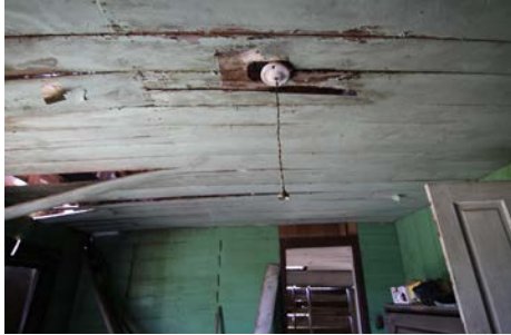
Ceiling in Living Room (looking south)
