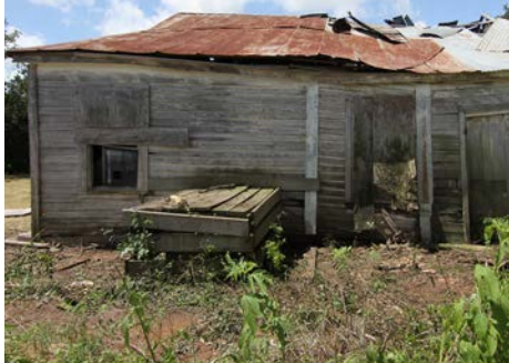
North Elevation (view of rock cistern)
