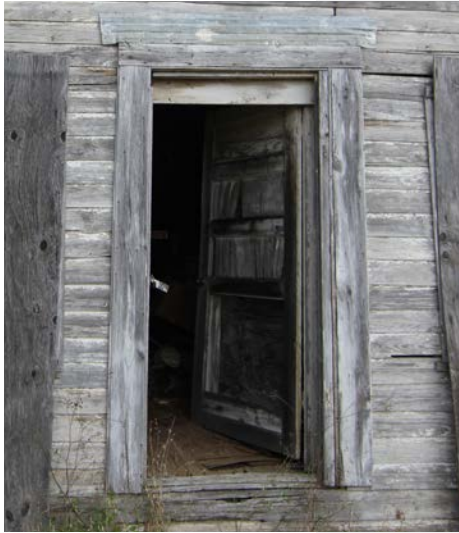
East Elevation Door
