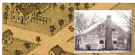
Figure 2. Photograph of Mina-Bastrop House Source: John Holmes Jenkins III, Ed, Recollections of Early Texas: The Memoirs of John Holland Jenkins . Austin: The University of Texas Press, 1958, 135-136.
