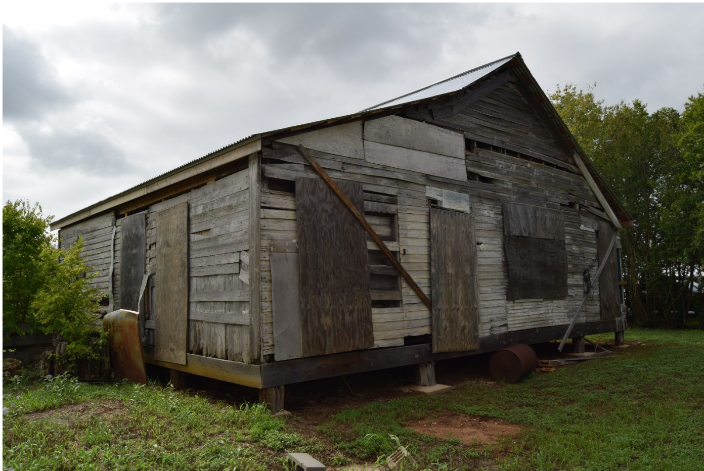
Photograph 8. North and west façades. Camera facing southwest.
