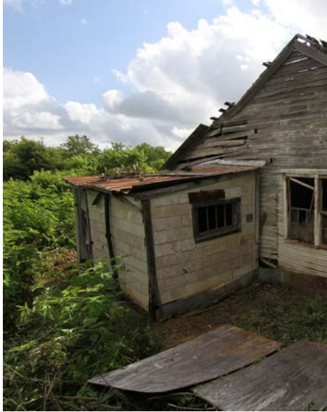
Kitchen/Bathroom Addition (looking northeast)
