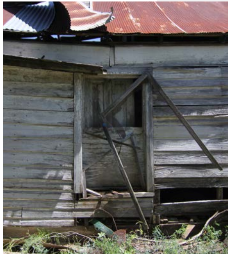
Low 6 Over 6 Window on South Elevation
