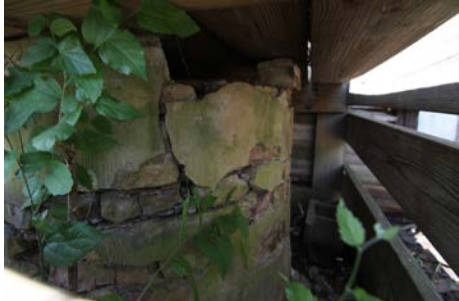
Detail of Rock Cistern (looking west)
