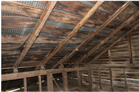
Roof Construction (looking northeast)
