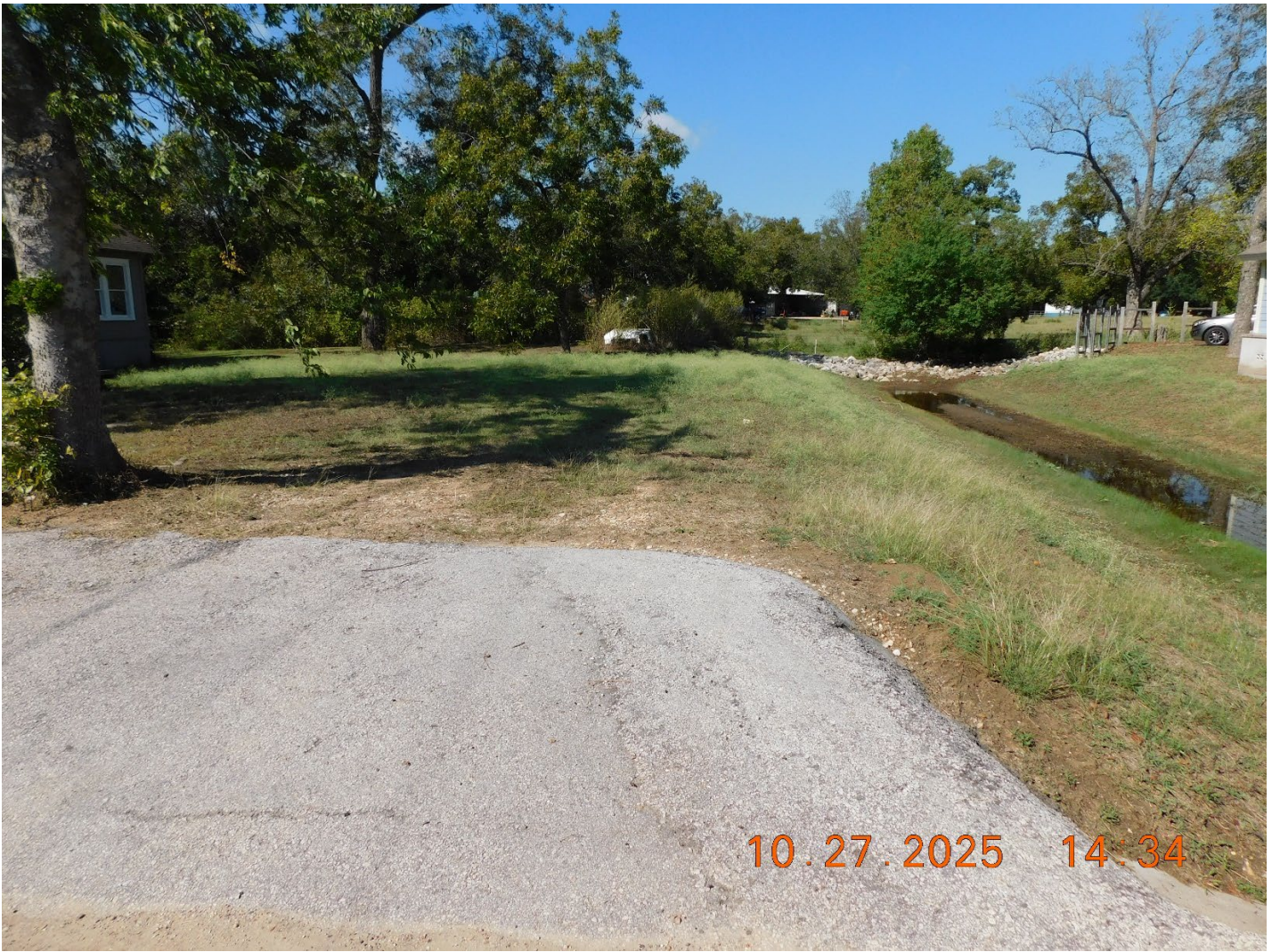
Photo showing Drainage Structure proximity to driveway.
