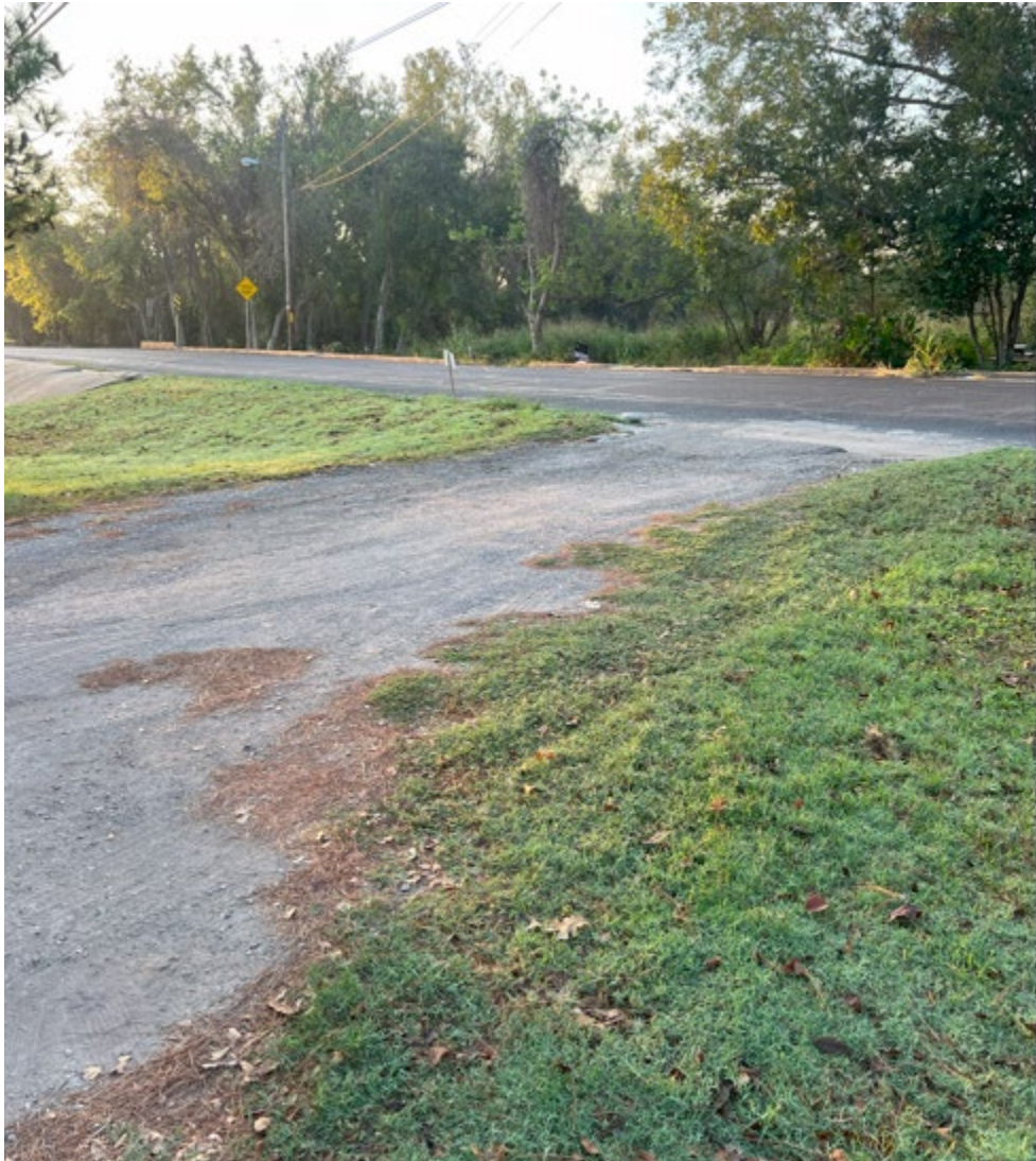
Photo showing the driveway connection to the road
