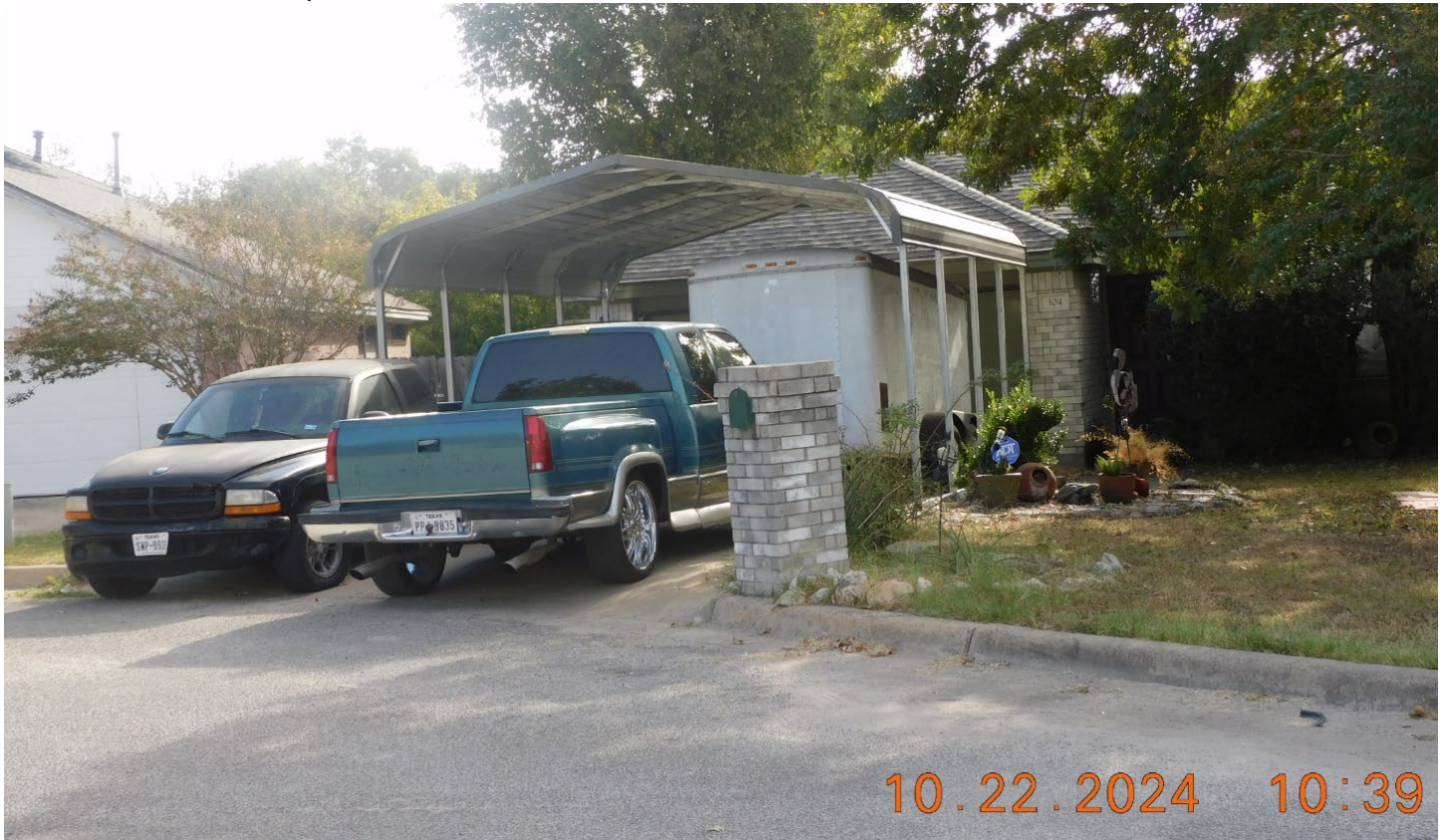
Photo #2 shows the detached 17' X 20' metal carport which was installed sometime between August 21 st and September 4 th .
