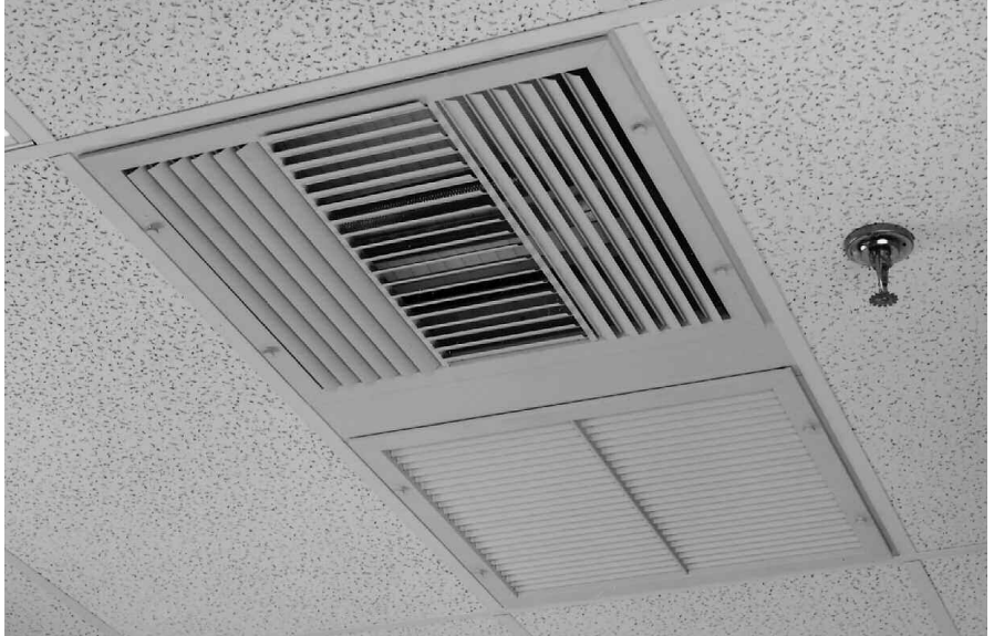
MC-880 in a T-bar ceiling system.
