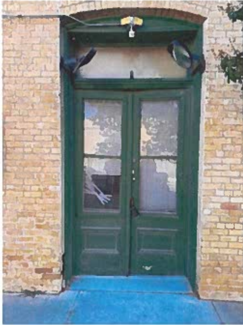
B3: Current Images of Side Doors (West)
