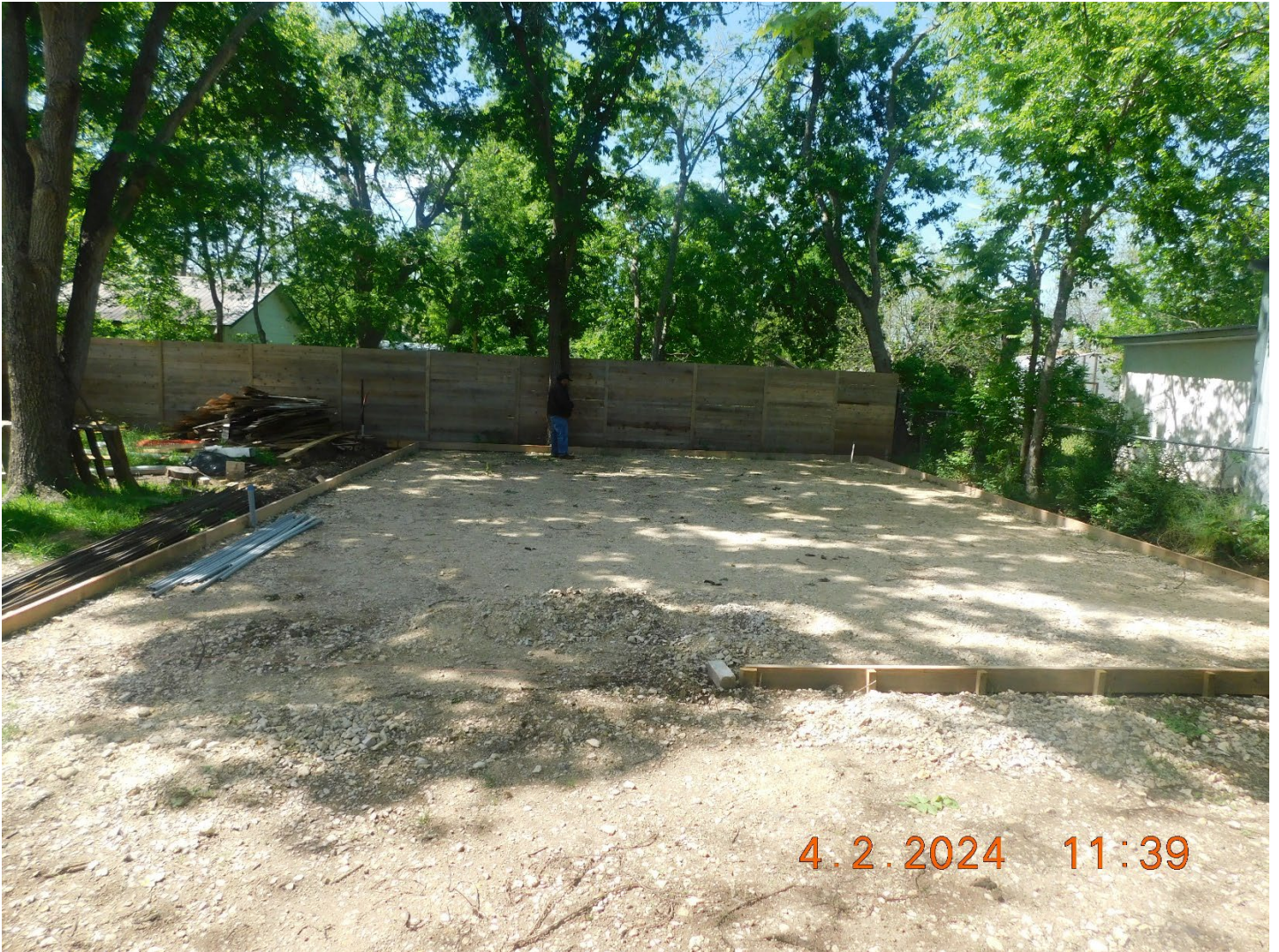
PHOTO # 1 – VIEW FROM FRONT OF PROPERTY TO REAR
