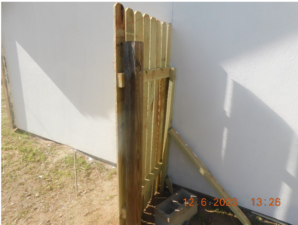
Gate at front on the east side.
