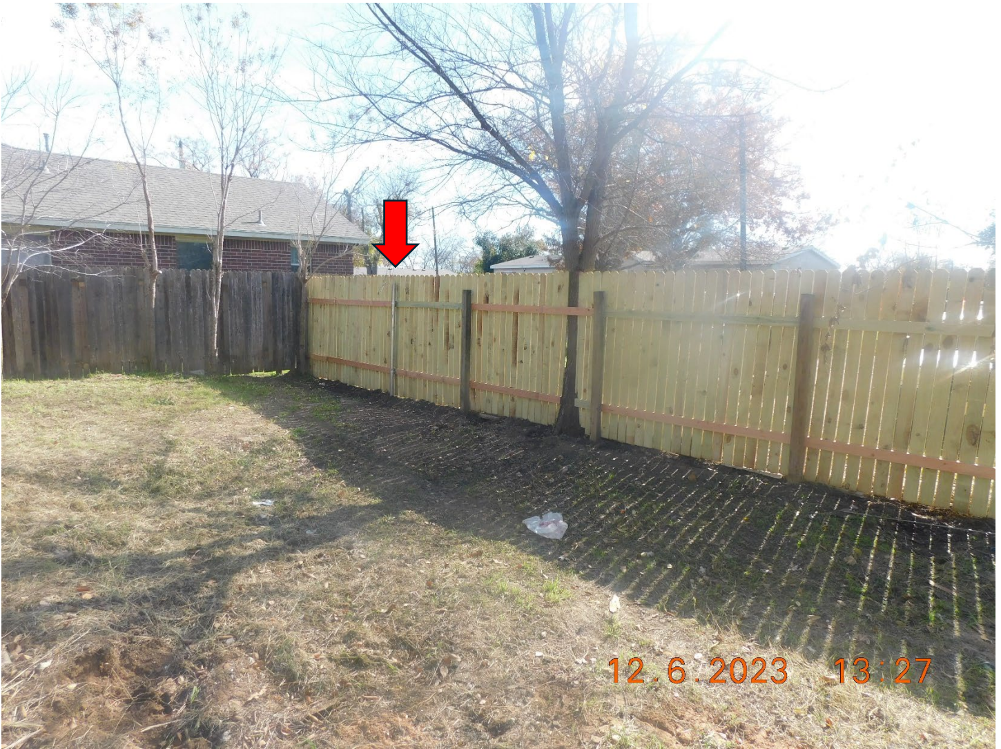
Mr. Alvarado placed a metal post in an area where there had been a gate in the far corner next to his neighbor to the east.
